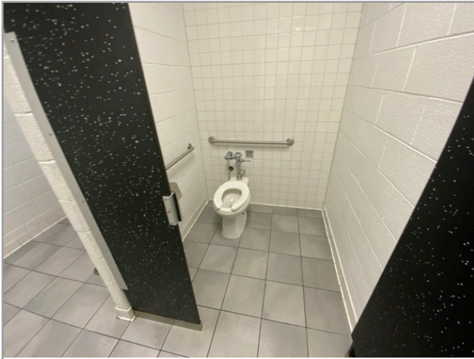
TOILET STALL OVERVIEW
