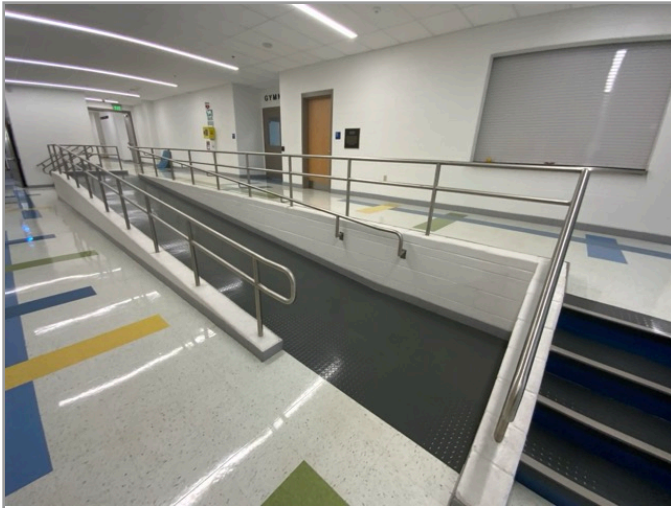
ACCESSIBLE INTERIOR RAMP
